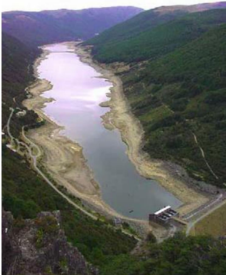
The Cobb Reservoir during the 2000-2001 summer drought. The power scheme has an operating water level range of 13.7m and the level at this time was 794.25m asl., just below the minimum operating level. The dam prevents movement of fish into or from the reservoir. (Photo courtesy of Georgina King, Environmental Management Services Ltd, Napier, 2001).
